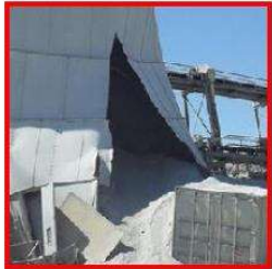
SILO RUPTURE
