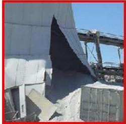
SILO RUPTURE
